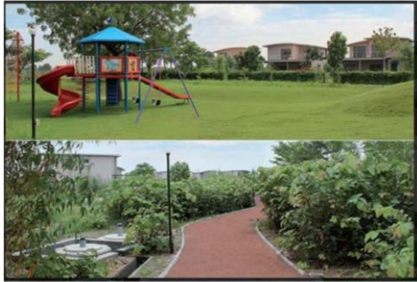
129 Weekend homes, Rancharda, Ahmedabad : Rainwater harvesting systems developed as part of society landscaping
