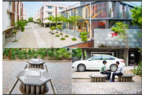
78@Gokuldham, Residential society, Ahmedabad : Rainwater harvesting systems developed in alignment with storm water management system
