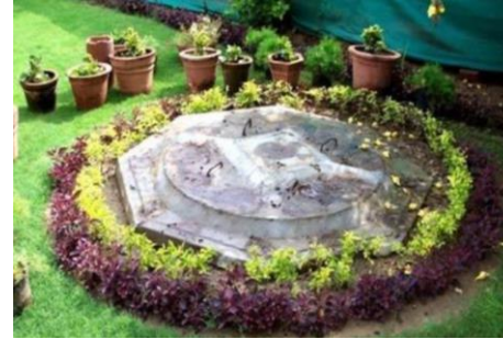
Parikh House – A resident of Ahmedabad city : Rainwater harvesting systems along ground water recharge structure (recharging existing bore well); water used for drinking purpose
